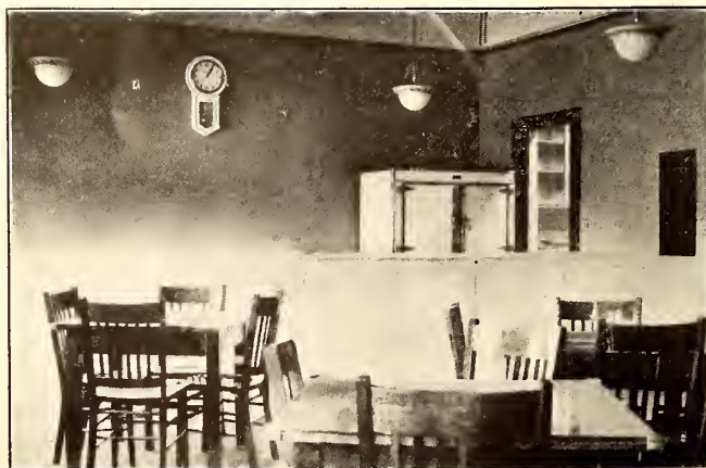
MILWAUKEE CARHOUSE AND STATION—RESTAURANT ON MAIN FLOOR OF TRAINMEN'S BUILDING
